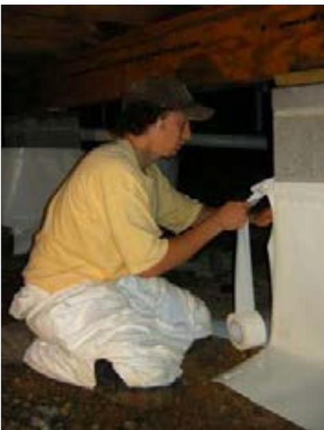
**Step 15** - Install material around all columns and piers. Material must be a minimum of 12' up piers. Use adhesive around perimeter of the column or pier and use vinyl tape to seal the seam. Apply adhesive with a bead that is approximately 3/16" of an inch in diameter. See Photos on Pages 8 and 9 for an illustration of a properly wrapped pier.
