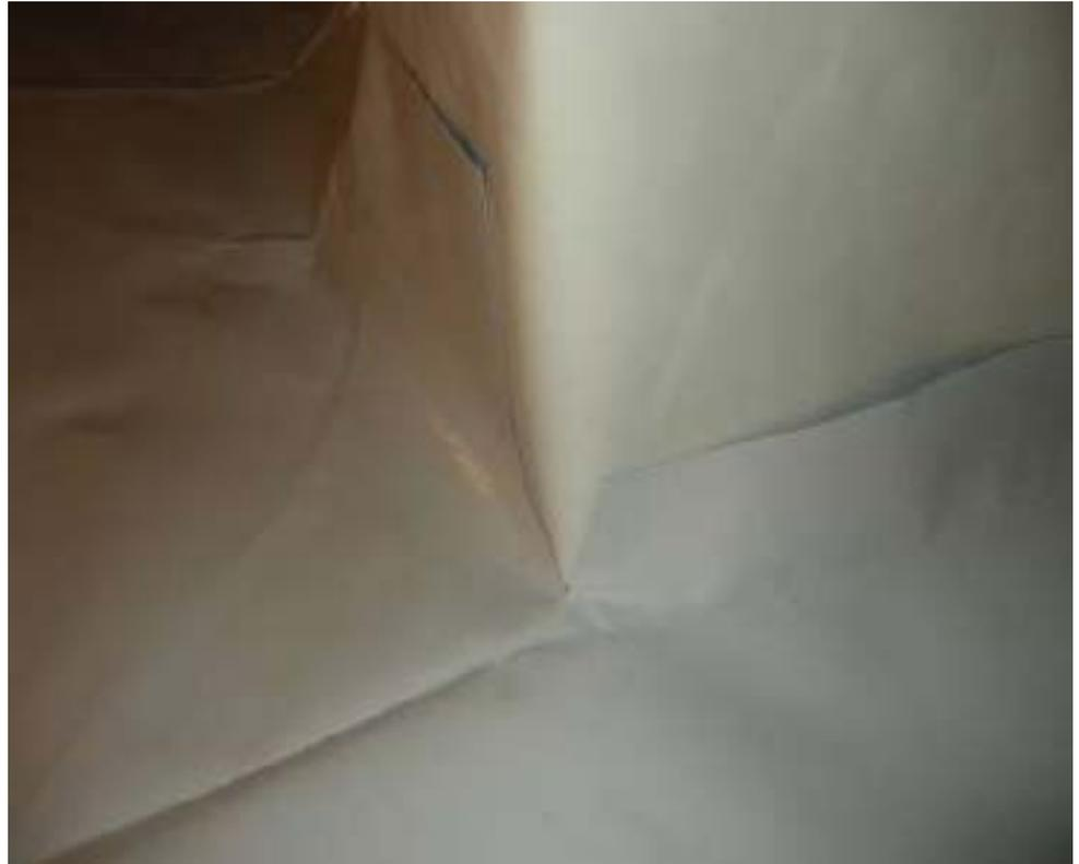
**Step 18** - Insulate band joist with minimum R13 fiberglass batt insulation or per your local code. Putting insulation in the rim joist is very important.
