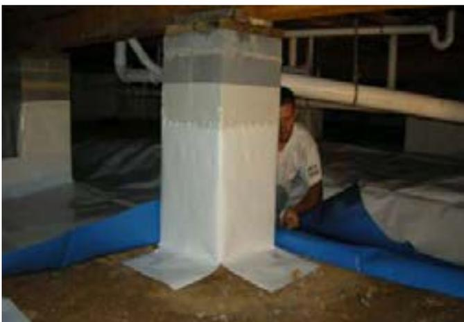
**Installing the Floor Material Around a Pier.**
